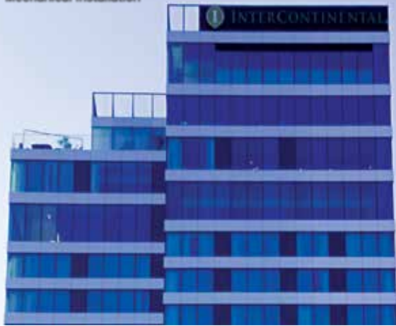
Hotel Intercontinental - Mechanical Installation
