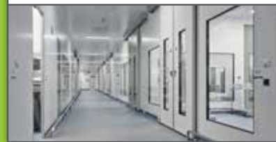
Cleangrad - Pfizer NEW New fire safety windows according to GMP standards.
